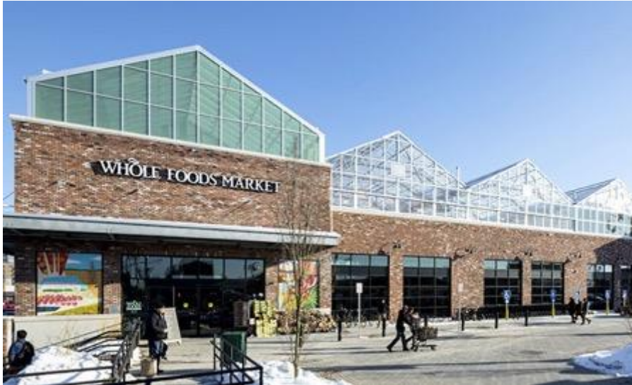
Figure 14 - Gotham Greens installed a rooftop greenhouse on top of a Whole Foods Market store in NYC.
